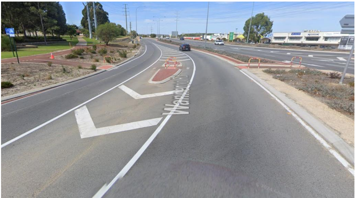
Figure 5-5: Example of Splitter Island on a Roundabout Departure Leg, Wanneroo Road, Tapping (source: Google Street View)
