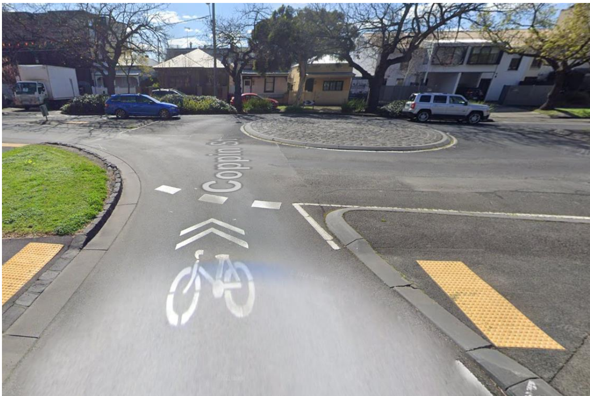
Figure 5-6: Example of Sharrow Pavement Marking, Coppin Street, Richmond (source: Google Street View)
