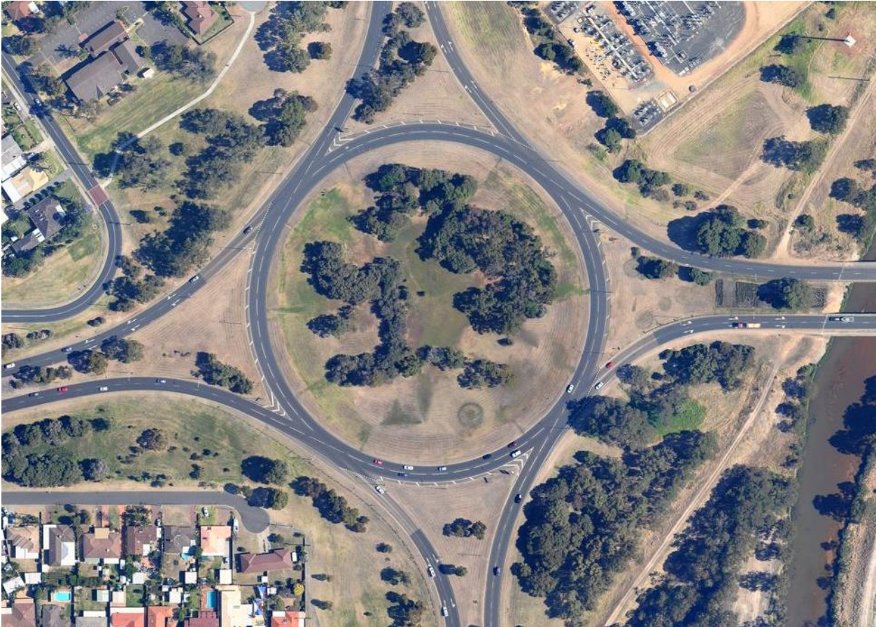
Figure C.1: Eelup Rotary in 2011 prior to Upgrading
