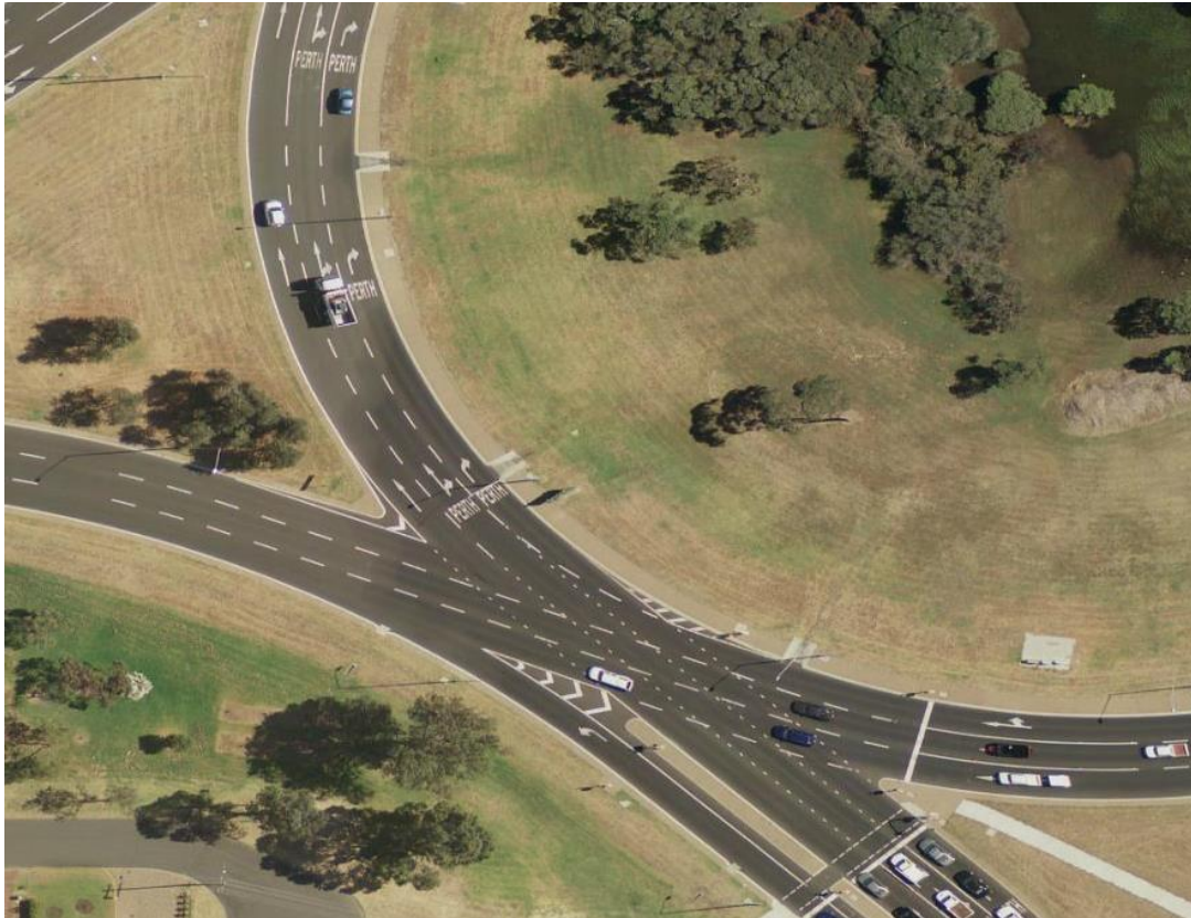
Figure C1.4 Example of Spiral Markings on a Signalised Roundabout in Bunbury
