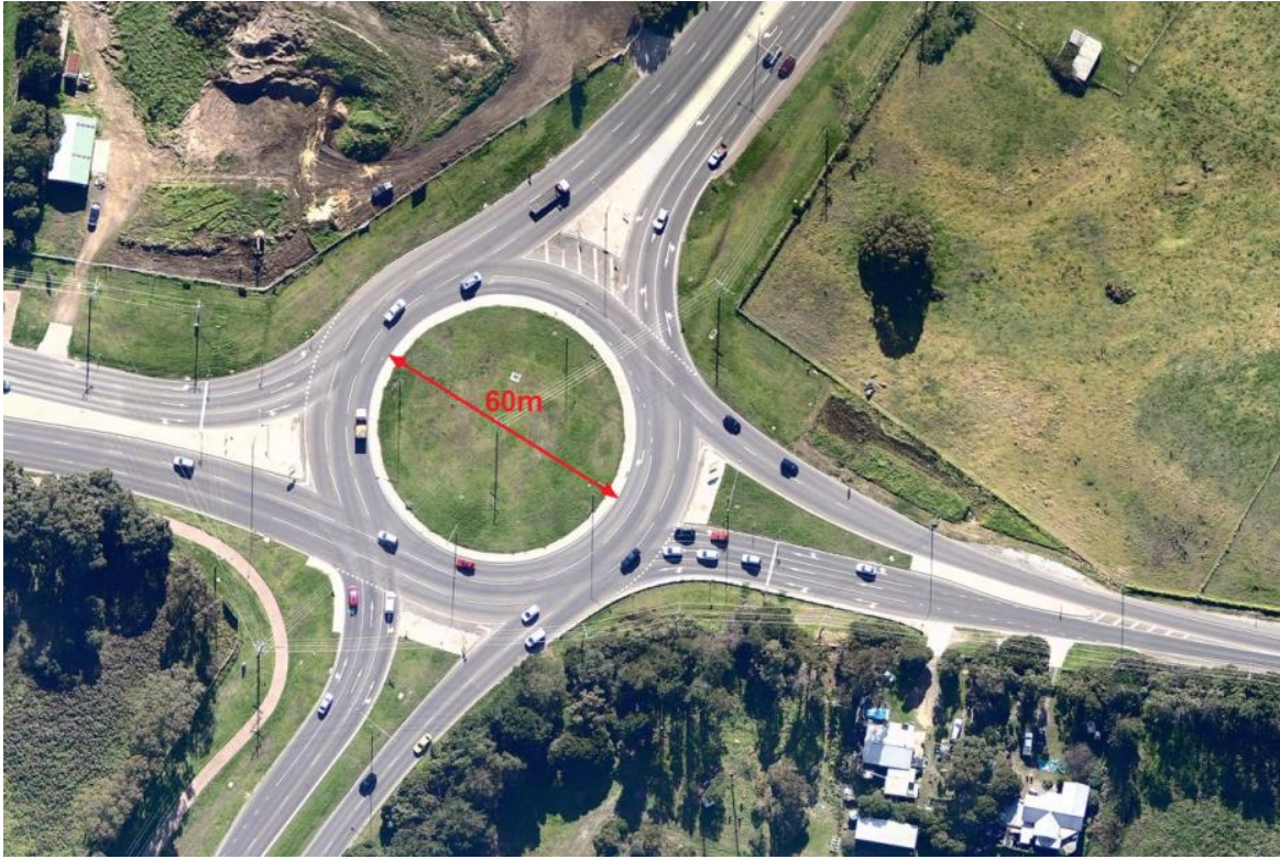
Figure B.1: Example of 3-lane Roundabout in Victoria (Dandenong-Frankston Rd (Dandenong Valley Hwy) / Thompsons Rd. Carrum Downs)
