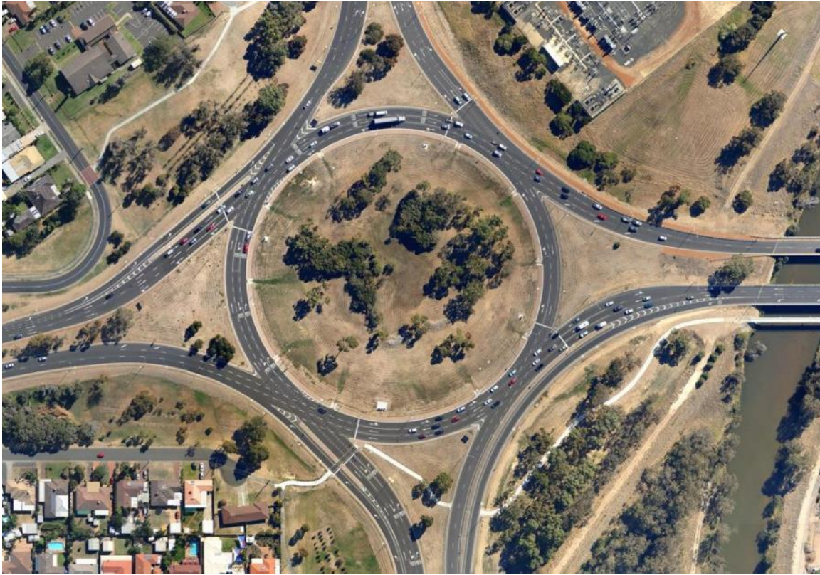
Figure C.2: Eelup Rotary in 2014 after Upgrading
