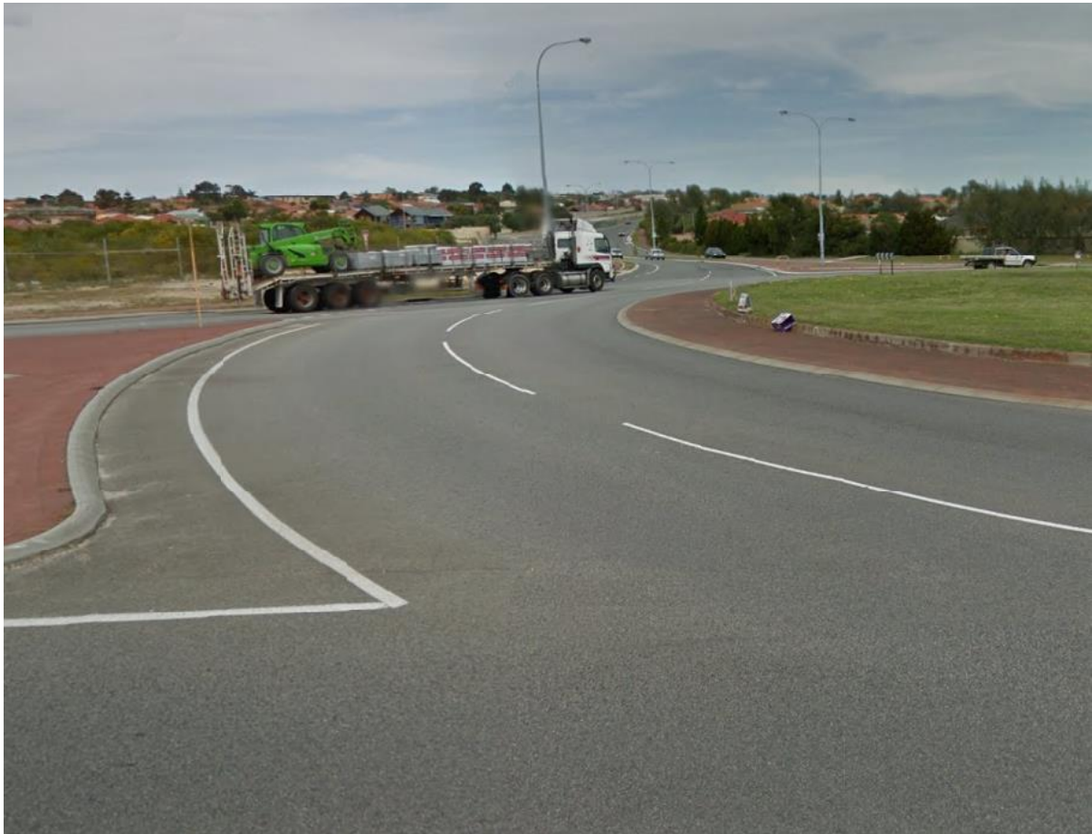
Figure 5-7: Example of a Heavy Vehicle Apron Around the Central Island of a Roundabout
