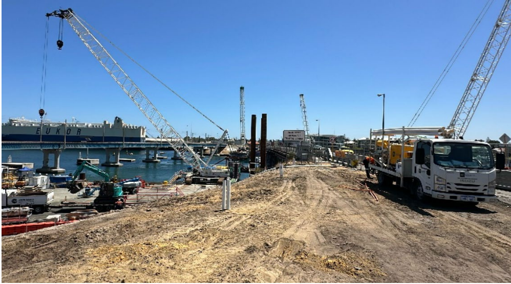
Figure 1: Abutment works on the southern side of the bridge in progress
