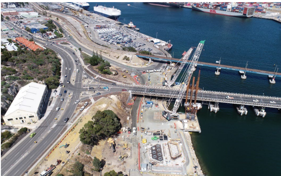
Figure 4: Aerial view of the southern construction area
