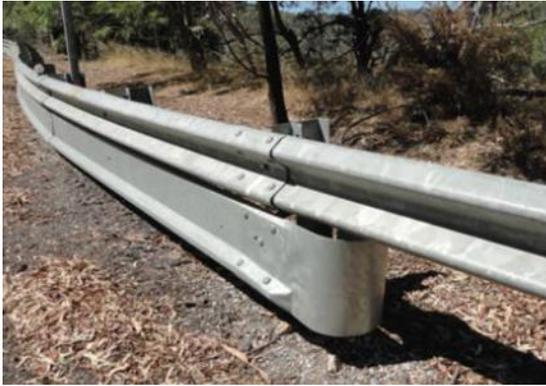
Photo 1: HIASA Rail Rolled End Section
